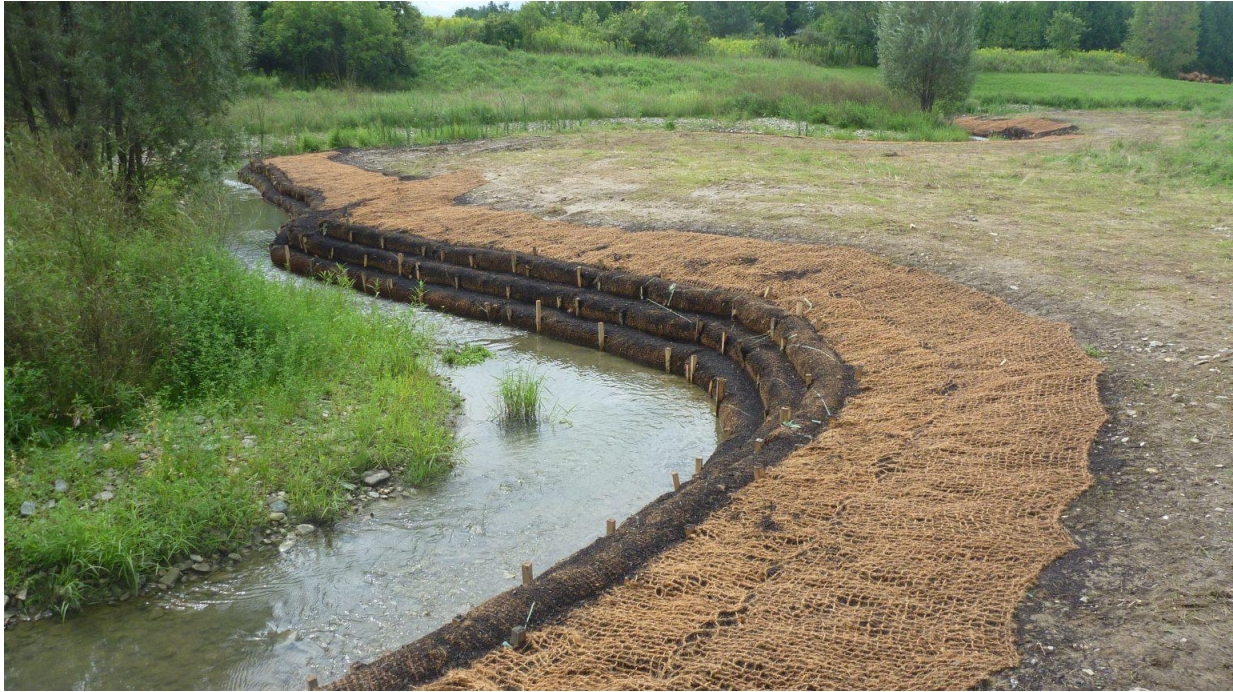
Example of Coir Rolls as bank protection
